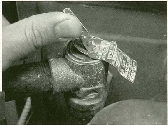
(Above) Lifting the handle of a pressure relief valve to check for proper operation
